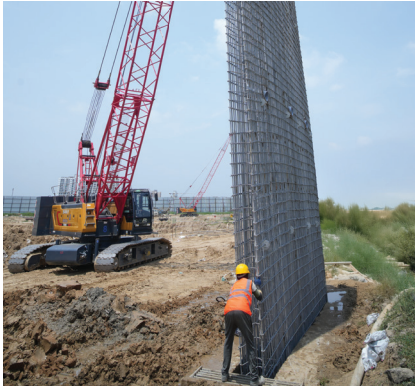
Diaphragm Wall/Retaining wall
