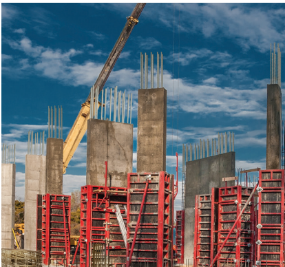
Columns and beams
