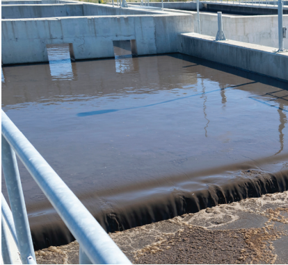
Sewage Treatment plant (STP)
