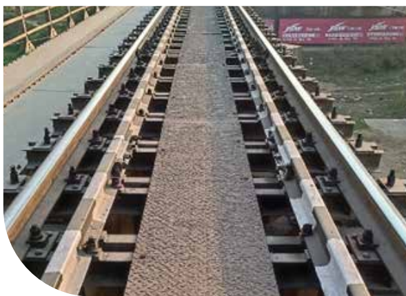
Revitalizing Nalhati Bridge, Eastern Railway – Howrah Division, West Bengal : Evolution from Corrosion-Prone Mild Steel to Enduring Stainless Steel Chequered Plates - Ensuring Longevity and Strength.
