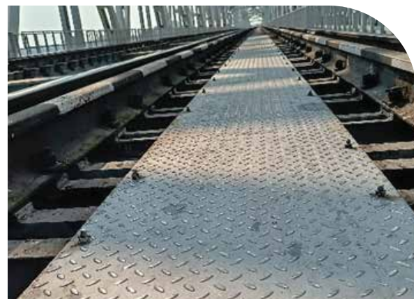
Transformation at Sampriti Setu, Eastern Railway – Howrah Division, West Bengal : From Corroded Mild Steel to Resilient Stainless Steel Chequered Plates - A Bridge to Durability and Reliability
