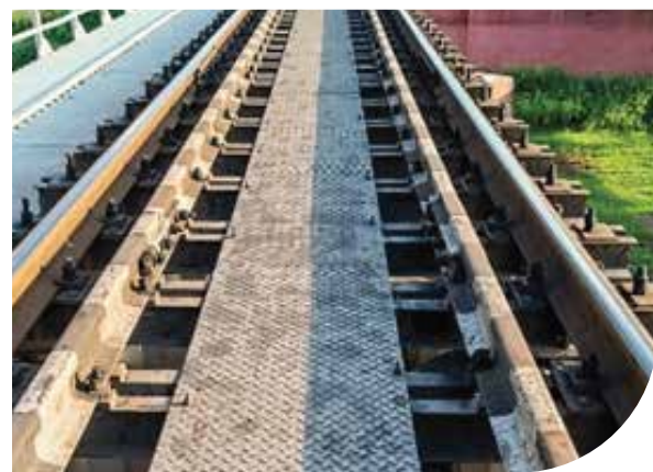
Revitalizing Nalhati Bridge, Eastern Railway – Howrah Division, West Bengal : Evolution from Corrosion-Prone Mild Steel to Enduring Stainless Steel Chequered Plates - Ensuring Longevity and Strength.
