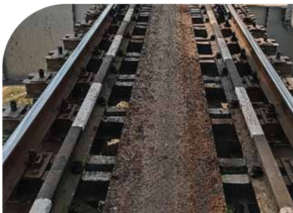
Transformation at Sampriti Setu, Eastern Railway – Howrah Division, West Bengal : From Corroded Mild Steel to Resilient Stainless Steel Chequered Plates - A Bridge to Durability and Reliability
